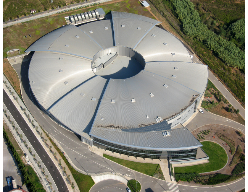
Alba Synchrotron Light Facility
