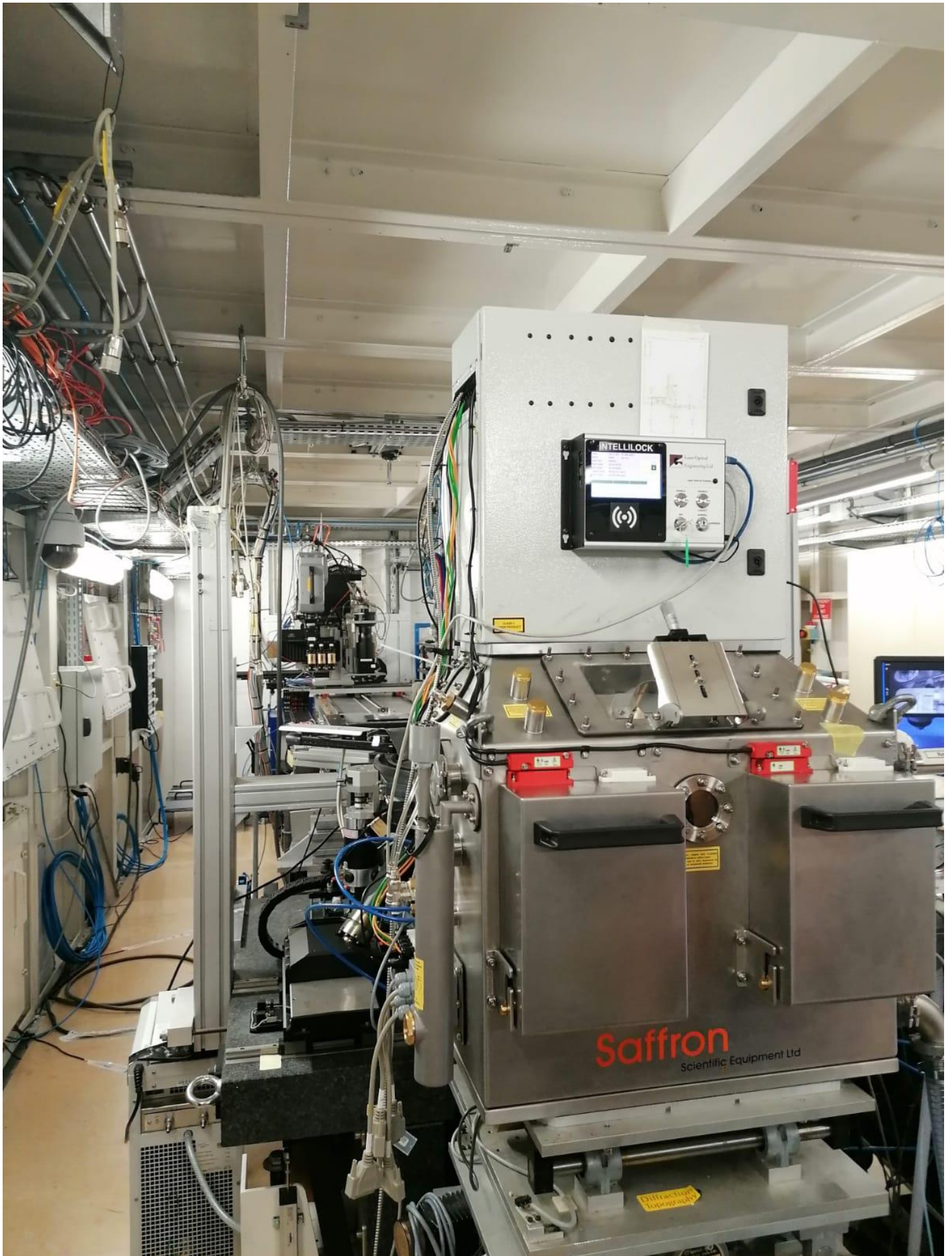
Figure 1. BAMPRII system mounted in ID19 hutch
